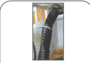
Crushed vent ducting, will impede proper and safe venting of fumes. Replace damaged duct
